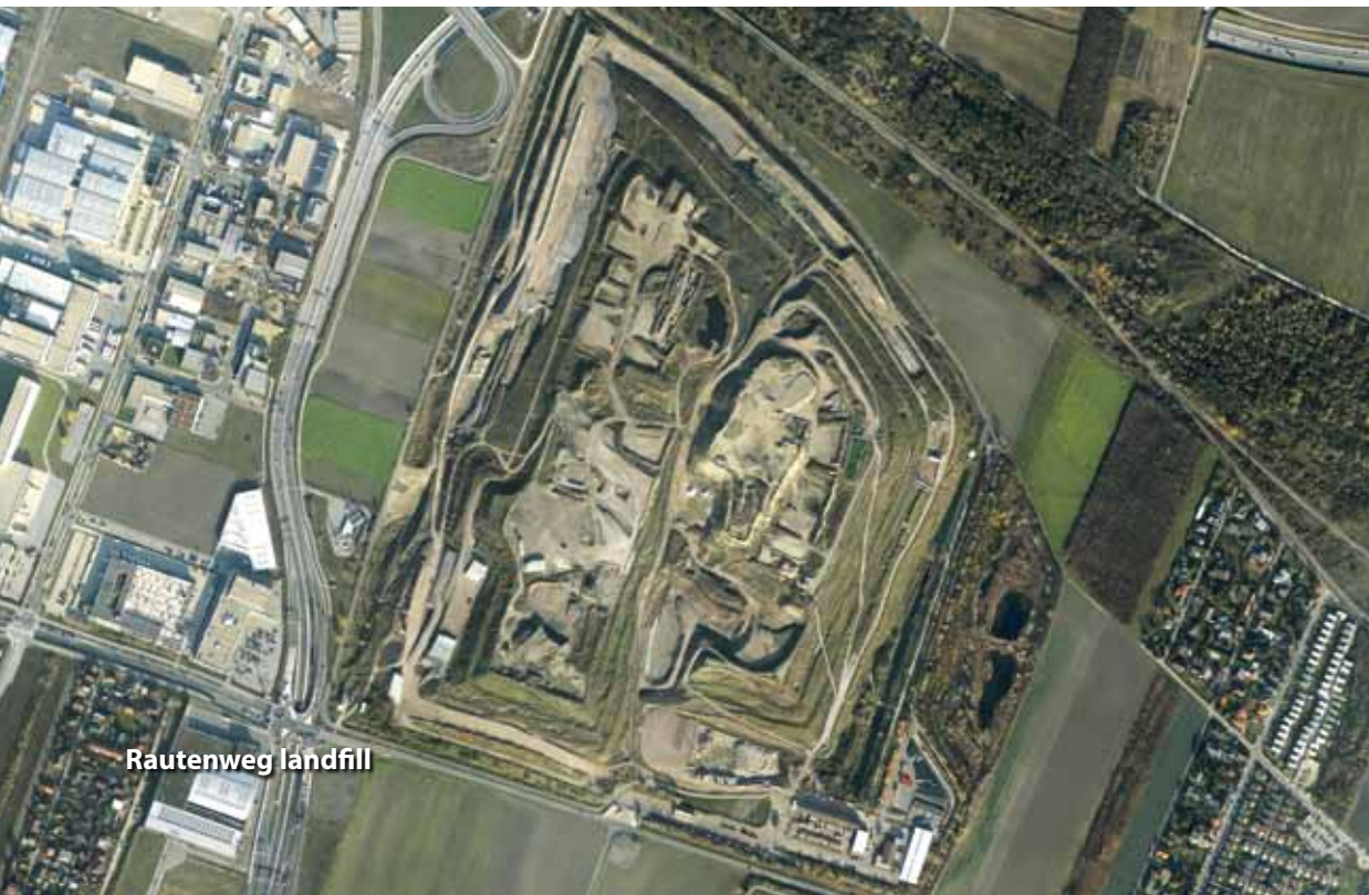
MVA Pfaffenau and Biogas Wien
